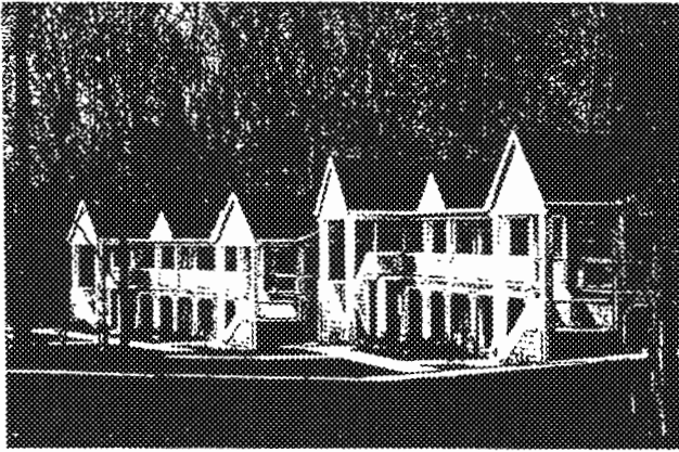
Housing for formerly homeless single mothers and children, developed with state funding assistance, West HELP, Greenburgh, NY. See p. 172
