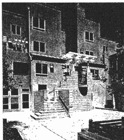
14. Dignity Housing, Oakland, California. Rear courtyard with children's play star
