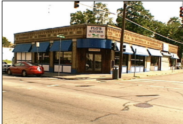
6. 3500 Burnet Avenue – Vacant business
