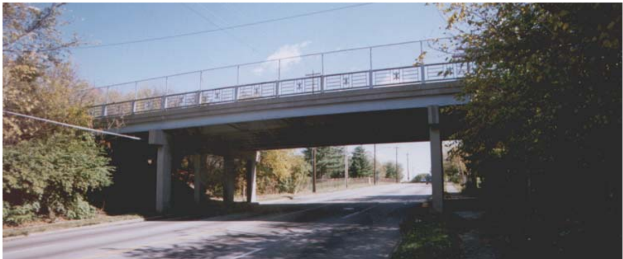
Figure 1. Decommissioned test bridge
