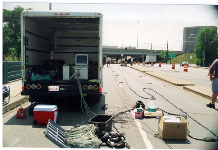
Figure 3b: VXI system and South test setup.
