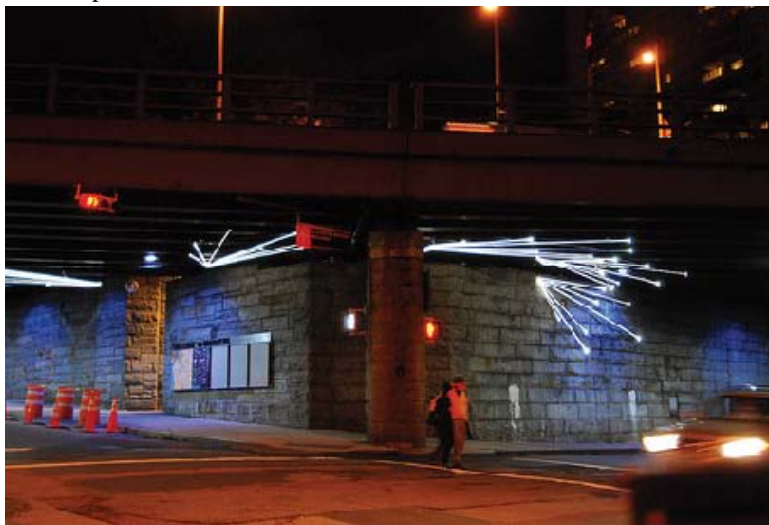
Lighting on an underpass can be an outlet for creative design as seen here in Brooklyn. Photo: DumboNYC.com
