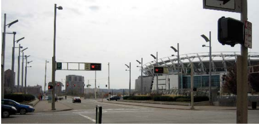
The overpasses across Fort Washington Way incorporate landscaped beds, wide sidewalks, and indirect lighting oriented to serve pedestrians and automobiles. Photo: Lauren Sullivan
