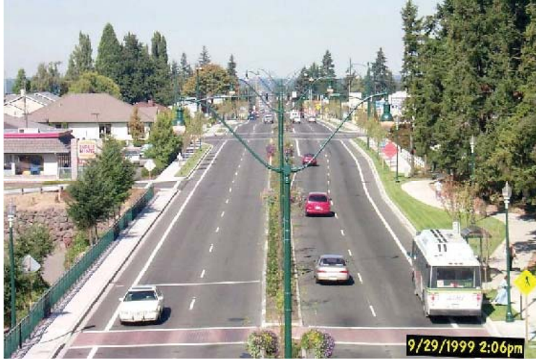
Bridgeport Way in University Place, Washington was transformed into a complete street. It incorporates auto lanes, bike lanes, sidewalks, bus shelters, crosswalks, a median, landscaping, and lighting for the road and the sidewalks. Photo: completestreets.org
