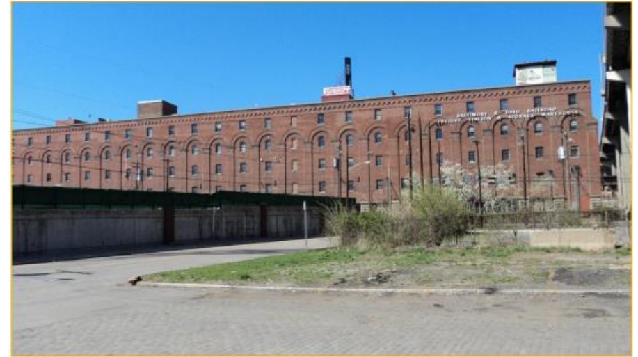
Photo 1: Longworth Hall - "Before" (The image above shows the east end of Longworth Hall "before" the introduction of the proposed Brent Spence Bridge Replacement/Rehabilitation.)
