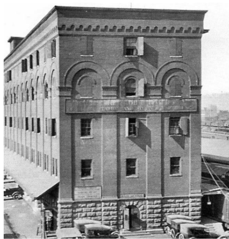
Original East Façade
